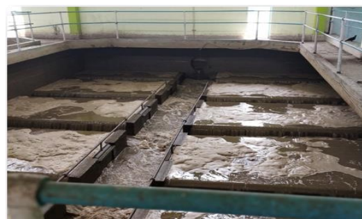
Figure 2 Rapid Sand Filter
